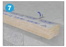
If the barrier is being used at the perimeter of a concrete floor slab, fit the barrier so it sits level with the top of the floor slab. Fold the clips over and secure them to the top of the slab.
