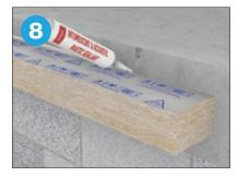
Check for any gaps between the barrier and substrates. All gaps should be fully sealed with fire rated intumescent mastic.
