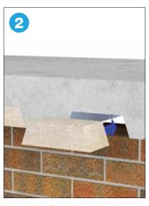
Fit the Fire Stop Block into the opening. It should fill the void completely. Any minor gaps or voids should be sealed with a fire rated intumescent mastic.
