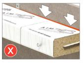
Insert three coarse wound screws through the intumescent and into the barrier. Once the façade is installed these should be wound out to touch the inside of the façade panel.
