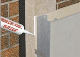
When installing more than one Closer, please ensure that the DPC tail overlaps the lower closer to ensure no moisture can reach the Closer.
