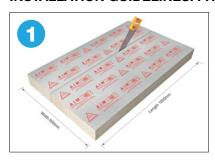
Measure the cavity depth and add 5%. Mark the slab and carefully cut using an insulation saw or hand saw. Please cut in the direction of the arrows printed on the foil facing. Note: This step is not required if installing Wall Cavity Fire Barrier cut to size.
